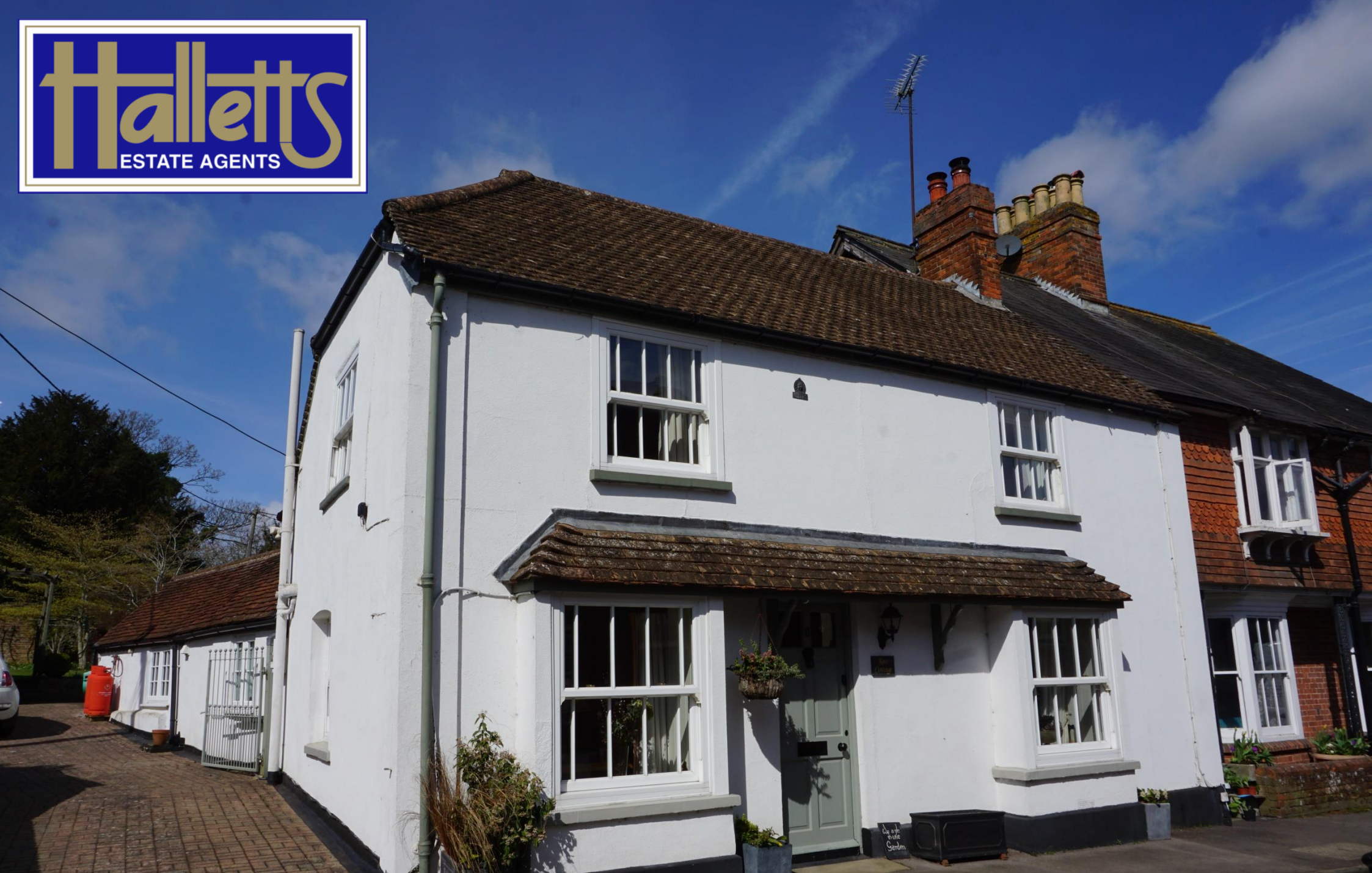
Rose Cottage 6 Church Street Kintbury Hungerford Berkshire RG17 9TR
